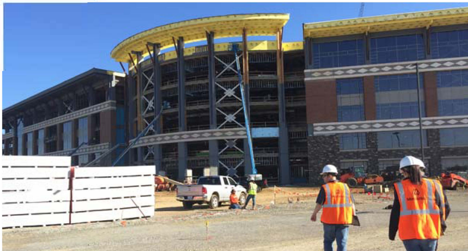
Workers walk toward the Choctaw Nation headquarters building under construction in Durant. (Courtesy photo)
