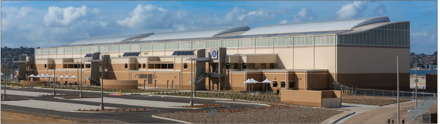
Naval aviation-themed entry elements that create a material and spatial hierarchy, and clearly delineate land-side points-of-entry help control the visual scale and disguise the industrial nature of the new three-squadron MH-60 Helicopter Maintenance Hangar at Naval Air Station North Island, Calif. PHOTOS BY HELIPHOTO.NET
