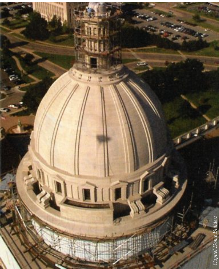
In this construction photograph, taken from the tower crane, the dome exterior appears to be nearly complete.
