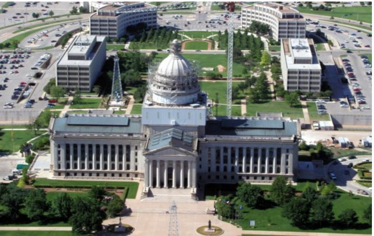
This construction photograph of the south facade of the capitol shows the scaffolding being removed and the temporary weather-resistant enclosure in place over the lower portion of the drum.
